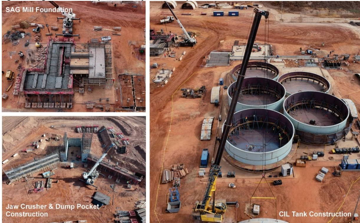
Figure 2: Stage I Hard Rock Expansion – Major Plant Component Construction
