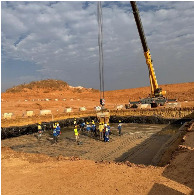
Figure 4: SAG Mill – Start of Raft Foundation
