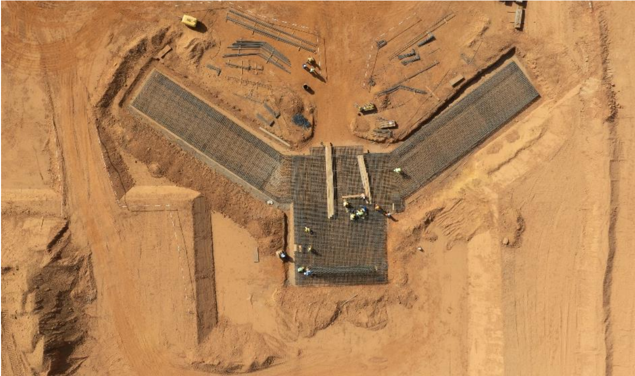
Figure 2: Dump Pocket/Jaw Crusher – Rebar Installation for Raft Foundation
