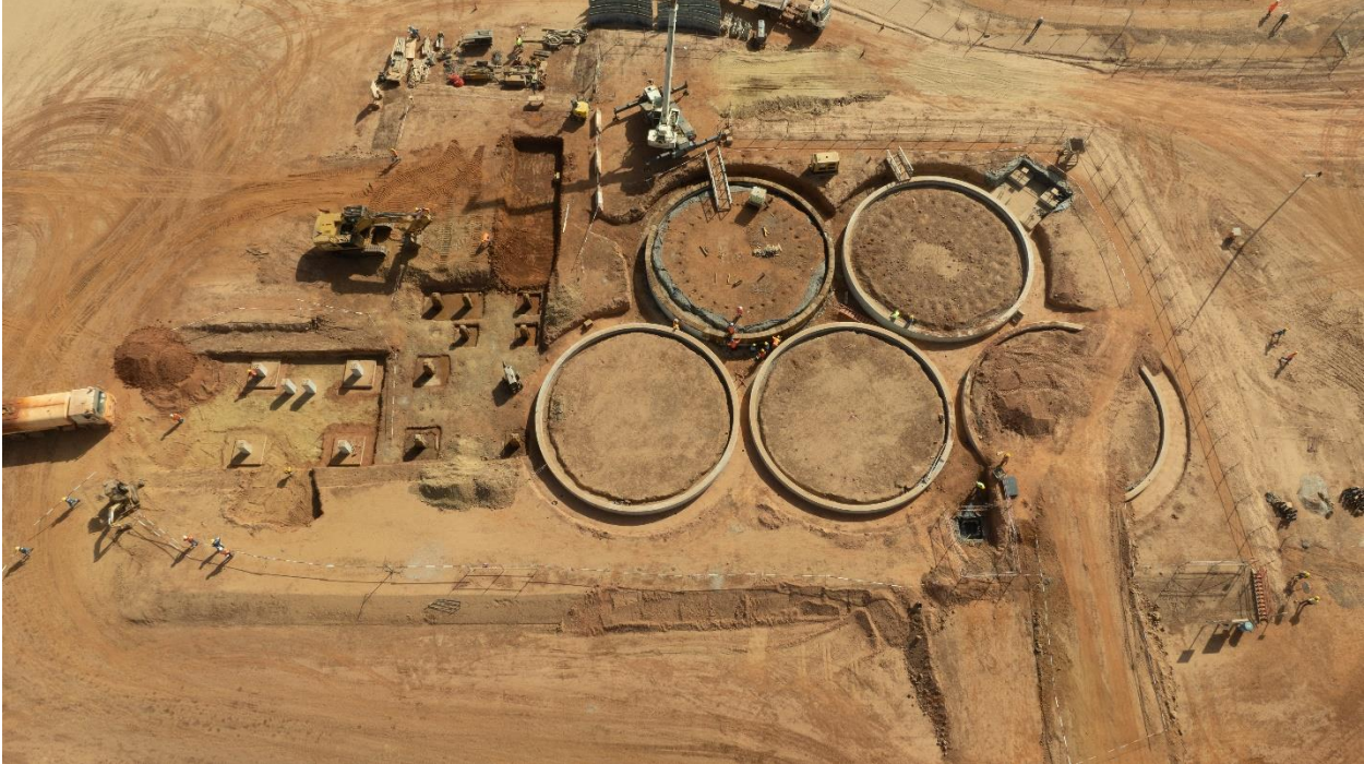
Figure 3: Installed CIL Ring Beams and Trash Screen Pedestals
