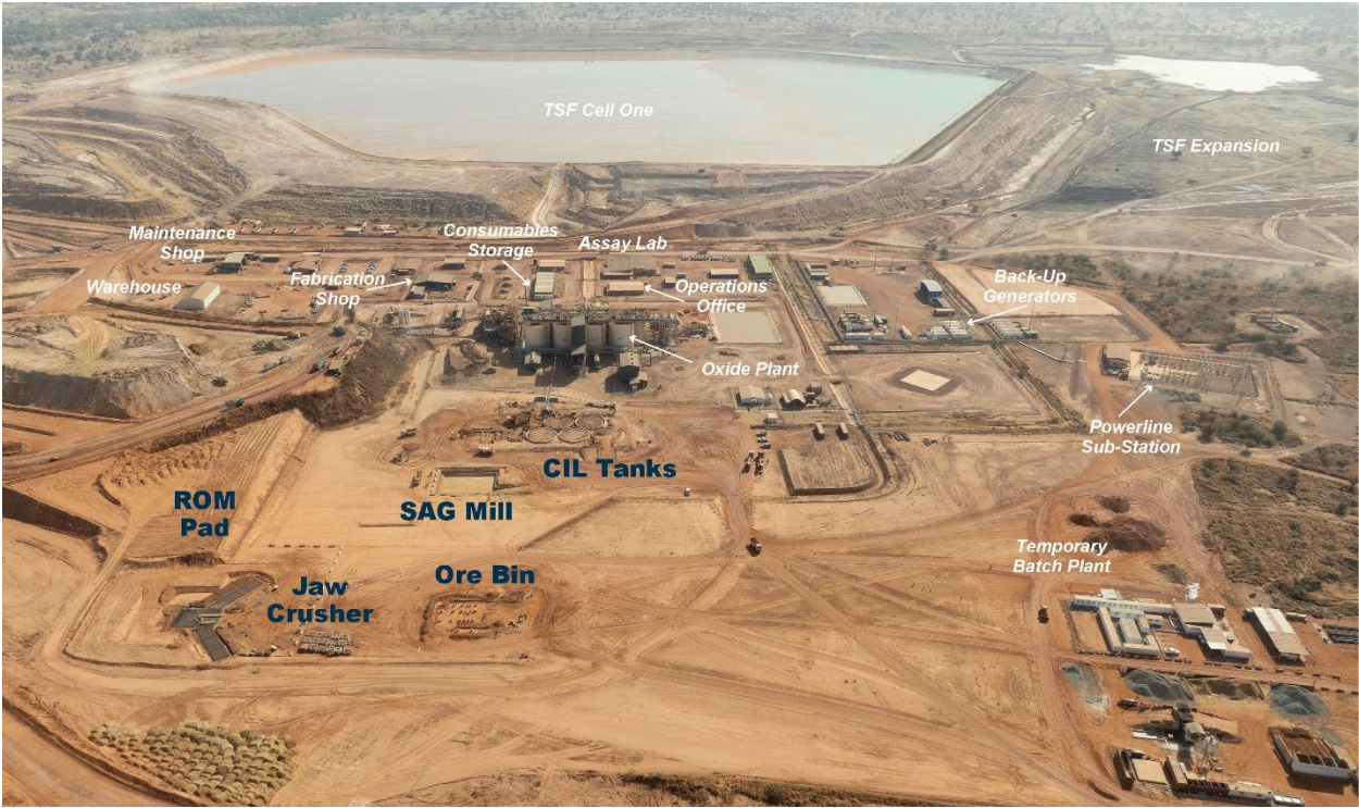
Figure 1: Bomboré Processing Complex – Hard Rock Plant Layout (blue labels) Relative to Oxide Plant and Other Established Infrastructure (white labels)
