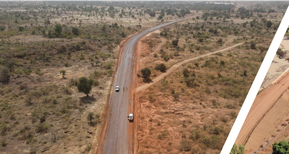
Main Haul Road
