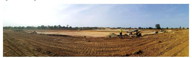
Figure 4: Surface Water Management Pond under construction
